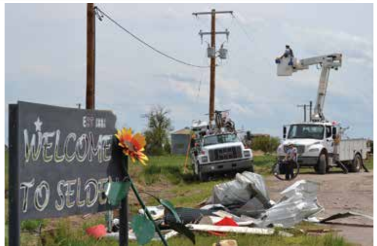
(Above) The Midwest Energy crew from Oakley makes repairs to powerlines near the local co-op in Selden, Kan., on May 24, after a tornado hit the town, tearing off roofs and damaging powerlines and gas meters.
