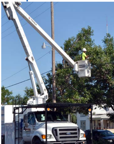
Chris Plante, Foreman with Solida Tree Service of Phillipsburg, trims branches away from lines in Hays. His crew trims trees from several miles of wire each week.
