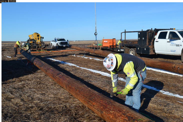
(Clockwise from Left) Linemen from Ward Electric cut through a pole with a chainsaw; (Above) An H-frame structure, dating to the late 1950s, is removed; (Below) A Ward Electric crew frames up one of 247 new H-frame structures along a 25-mile stretch of transmission line between Nekoma and Ness City.
