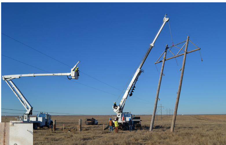
(Clockwise from Left) Linemen from Ward Electric cut through a pole with a chainsaw; (Above) An H-frame structure, dating to the late 1950s, is removed; (Below) A Ward Electric crew frames up one of 247 new H-frame structures along a 25-mile stretch of transmission line between Nekoma and Ness City.
