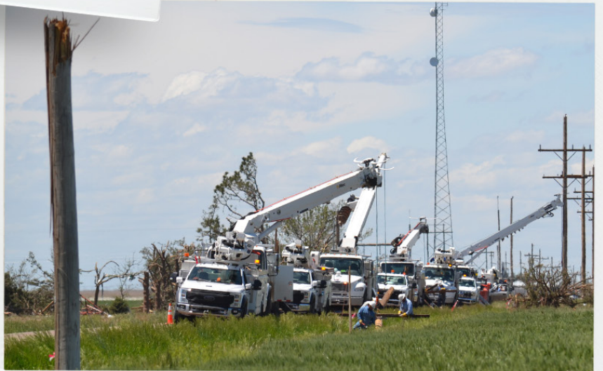
Restoring Power After Tornado in Grinnell, Kan.
